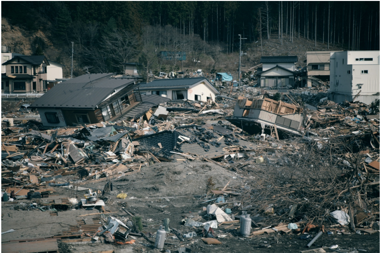
Figure 5: Tsunami damage, Fukushima, Japan, 2011
